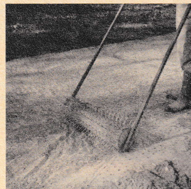
(5) A close-up view of the roller used to punch holes in the plastic. This one is home-made from a small log with nails imbedded in it.
