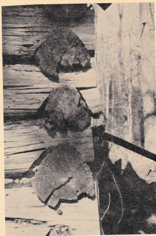
The end of a log tobacco barn showing the way the logs were notched to hold them in place. Using this method there was no need for nails to secure the logs.
